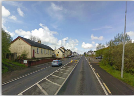
Plate 5-1: Existing N4 through Castlebaldwin
